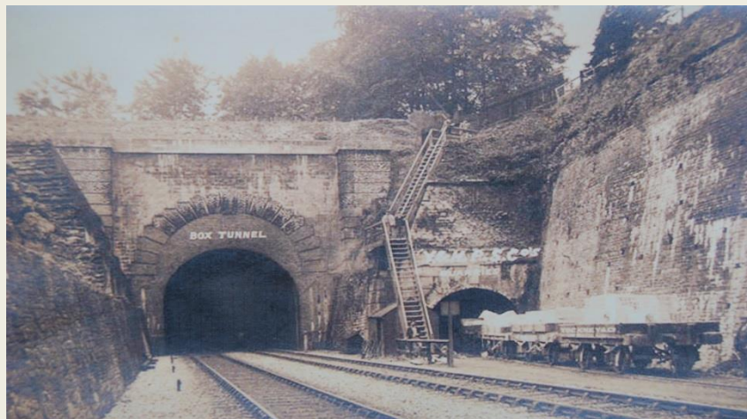
Box tunnel April 6 th 1904—we can just see the 'light at the end of the tunnel—low centre'
