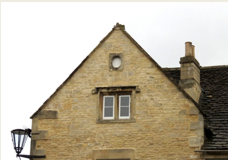
Above: flank wall with apex oval light and, below it, recessed mullion window with hood over.
