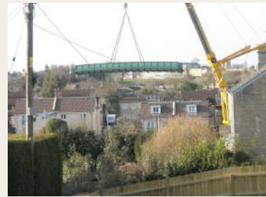
New footbridge being swung into place, photo by Robin Jackson
