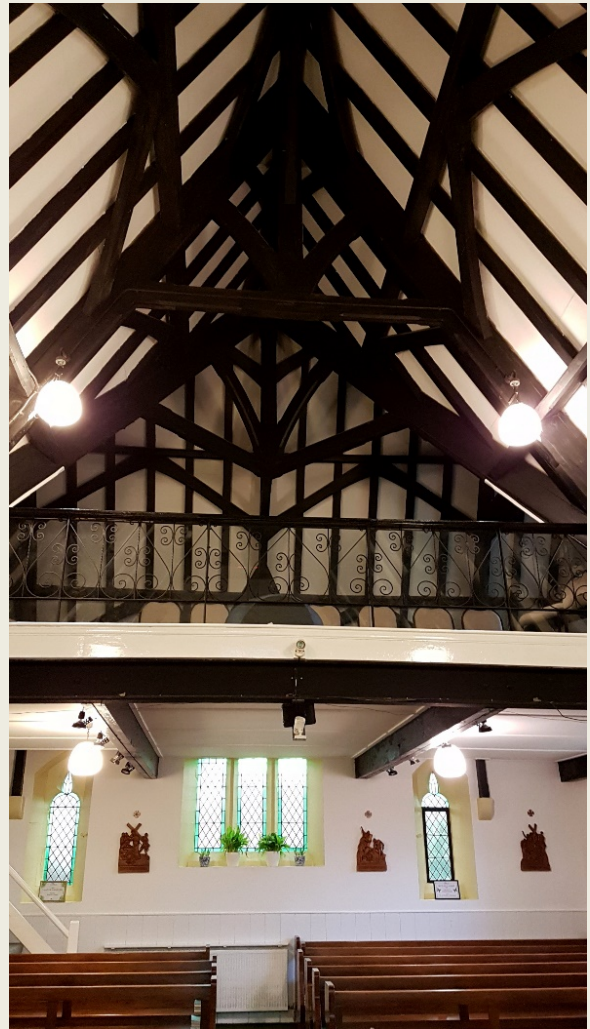
View of the main body of the former school and the gallery above.
