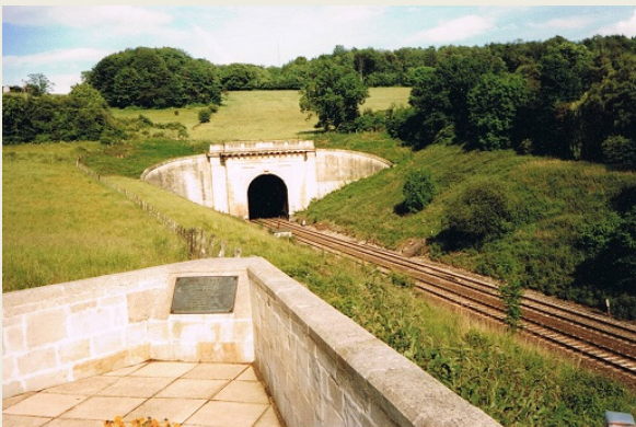
West end of Box tunnel c. late 1980s
