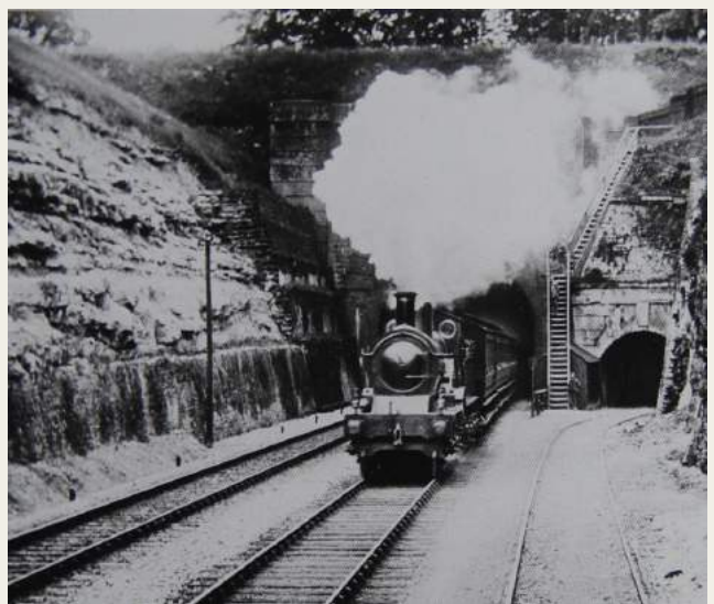
One of William Dean's famous 4-2-2 singles of the mid 1890's emerging from the Corsham end of the tunnel. The tunnel to the right gave access to the stone quarries of the Hartham & Yockney Stone Quarrying Company.
