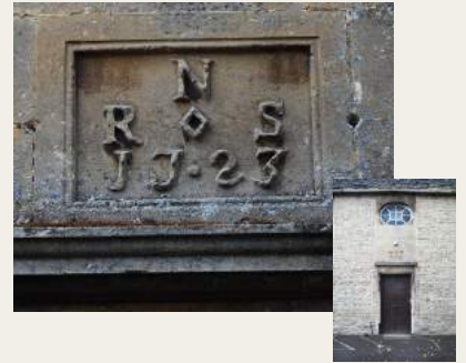
3) Mansion House Stables
