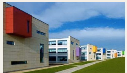
The new era MOD site at Basil Hill
