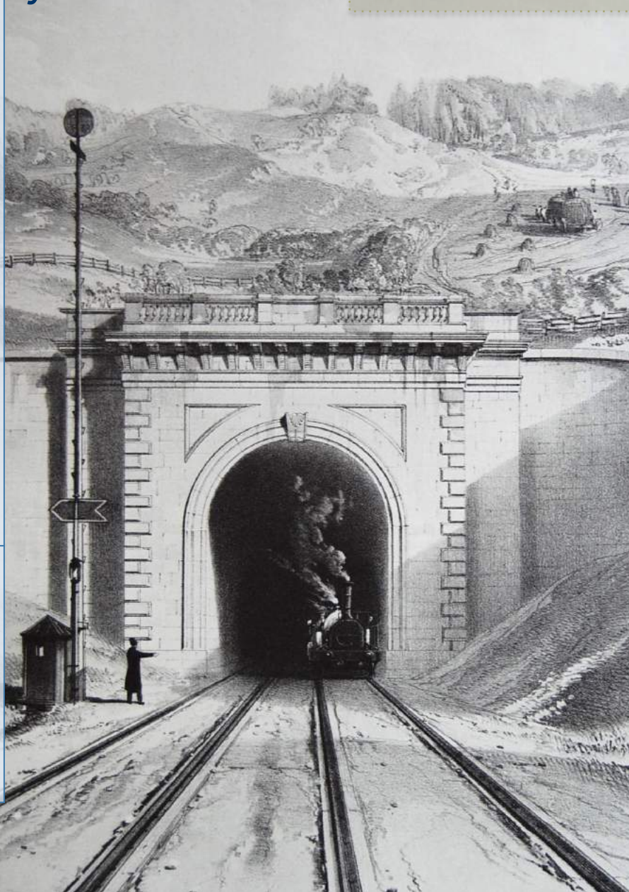
Train emerging from Box Tunnel, an engraving by John Bourne in 1846. Note the early signal on the right with its own 'signalman'.
